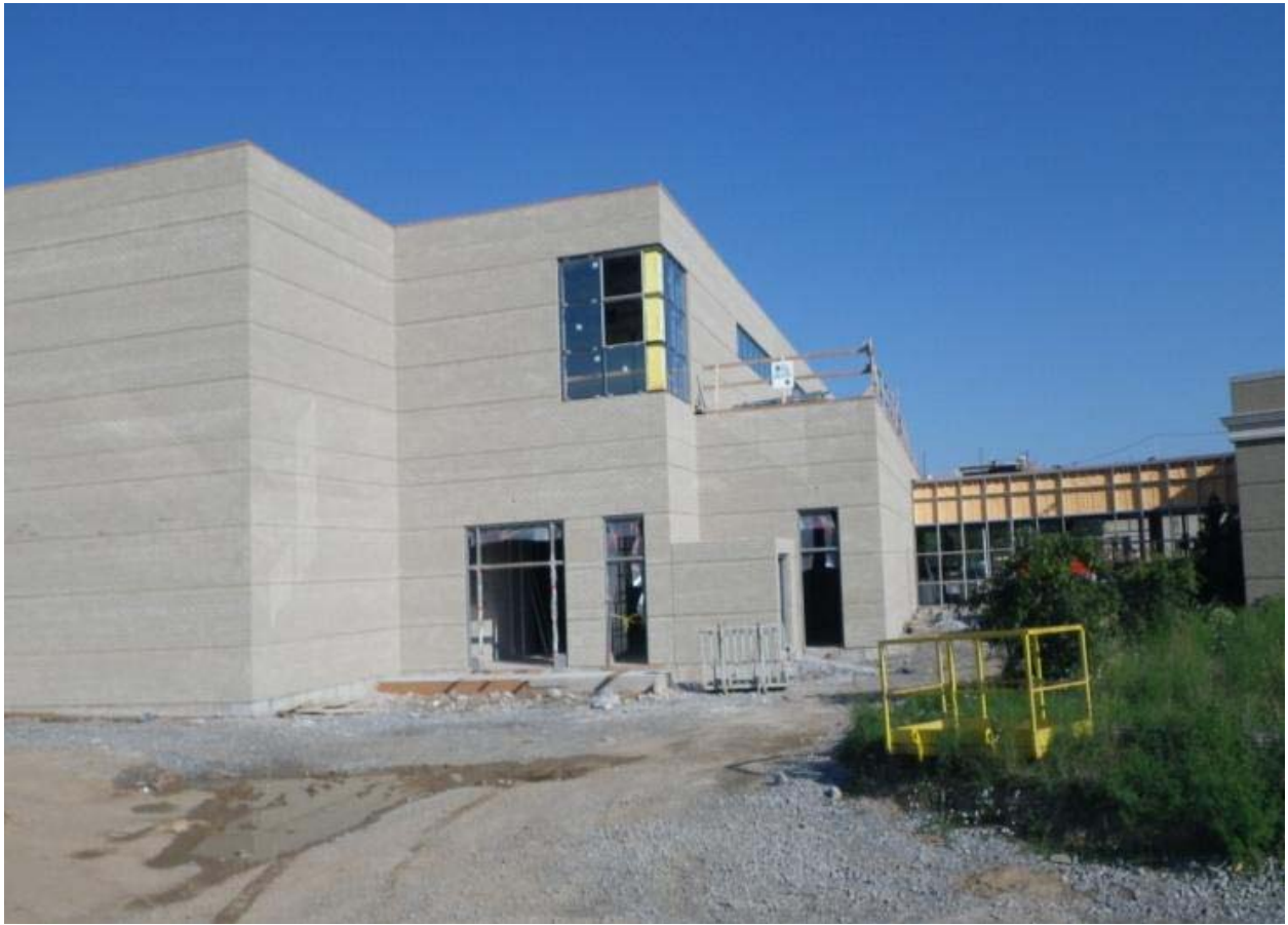
Glazing installation as viewed from back of back of building.
