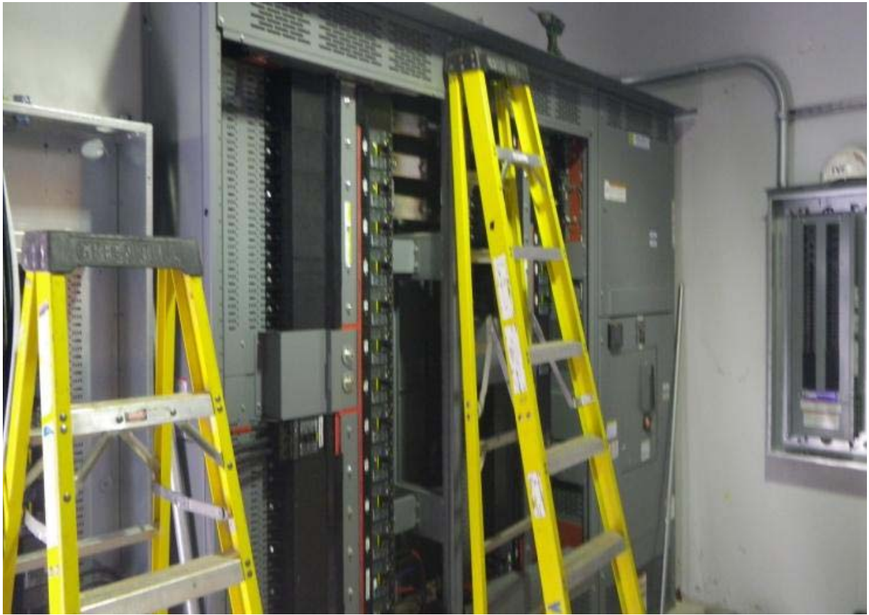
Switchgear installation.
