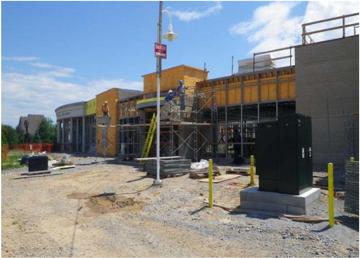
Window framing and masonry work proceeding at building entrance.
