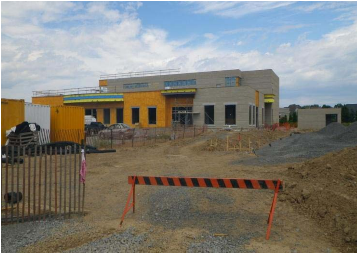
Brick progress on west elevation.
