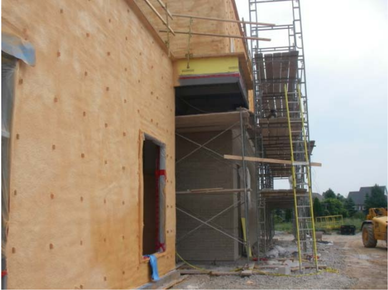
Brick and Spray Insulation South Elevation
