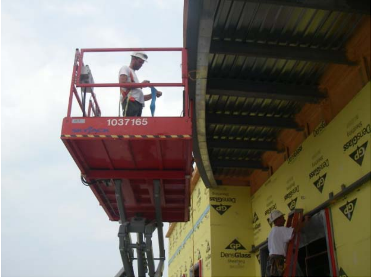
Sheathing west elevation
